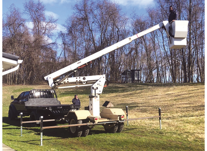
Hardman's lift has a 37 ft. working height and is rated for 350 lbs. with the boom extended.
