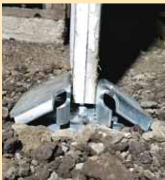
Concrete support post with foot plate keeps the bottom of large doors aligned.
