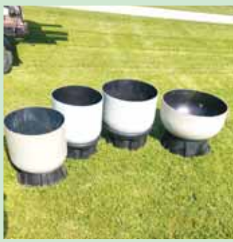
Fiberglass water pressure tanks are cut using a grinder with a cut-off blade.
