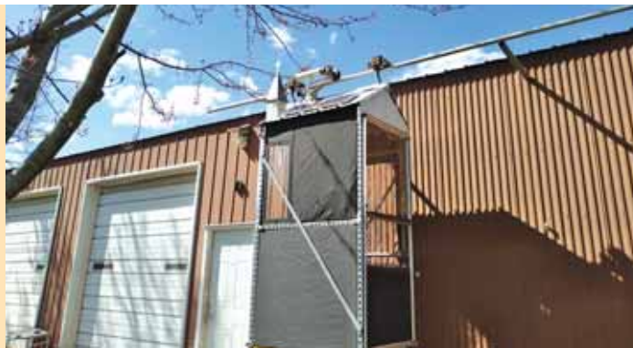
Altenweg used a discarded ice fishing house frame made from 1 1/2-in. wide, 12-gauge Unistrut hangers. It's covered in see-through vinyl panels with a roof of tin.
