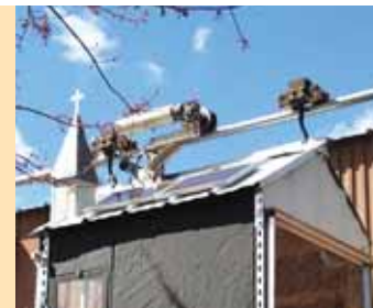
Altenweg used a discarded ice fishing house frame made from 1 1/2-in. wide, 12-gauge Unistrut hangers. It's covered in see-through vinyl panels with a roof of tin.
