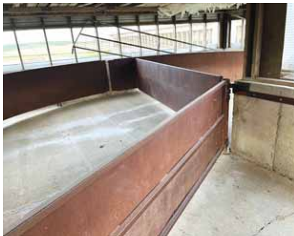
Guide panels swing on sturdy metal hinges while side panels are anchored to the floor and sidewalls.
