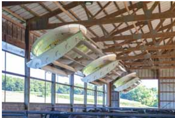
Arctic Blast fans use ultra-fine water particles to absorb heat and transport it away, so they can change the temperature fast without leaving a wet feeling in the room.
