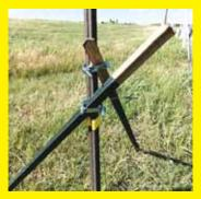
I make corner posts using three T-posts and U-bolts. I drive the braces into the ground and attach the tops to the corner post with either two smaller U-bolts or one big one. If the ground is really soft, I dig a 6-in. dia. hole around the brace postholes and surround with concrete. Really gets the job done. (Jack Griffith, Venus, Texas)
