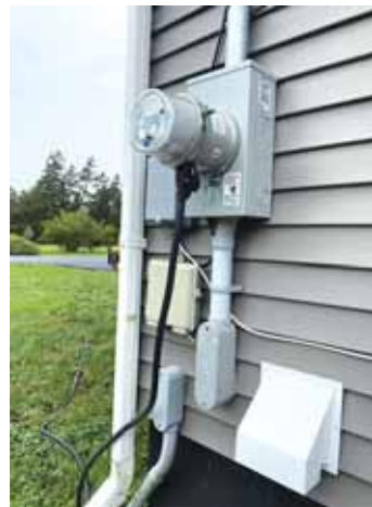
Langelier says the GenerLink is safer than other interlock switches as they protect generators and don't allow utility lines to back-feed.
