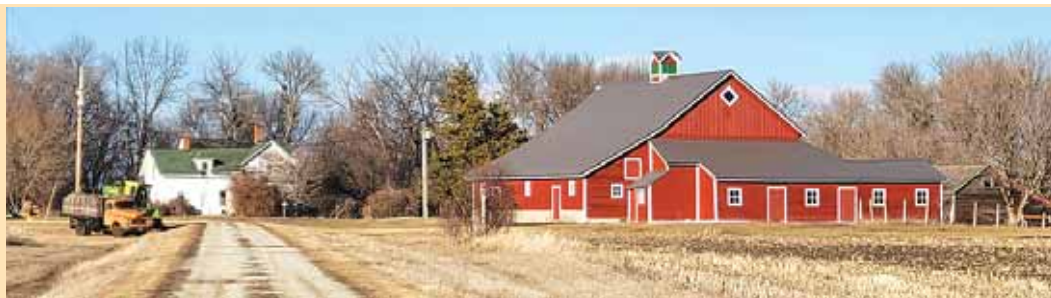
Rebuilt, reroofed, reinforced, and repainted, the unique thresher barn is once again an iconic red landmark on the Keeley farm near Janesville, Minn.
