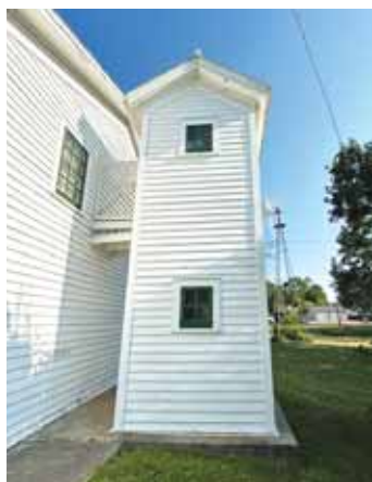
Each level has three holes. A wooden chute allows the waste from the top floor to go into the pit under the outhouse.
