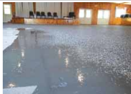
Polyurea base coat with vinyl flakes.
