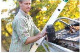
UV-protected, weather-resistant bristles are designed for all climates, from areas with heavy leaf fall to regions prone to ice and . snow. To install, simply slide each 3-ft. section of GutterBrush into existing guttersno tools, fasteners, or modifications are required.
