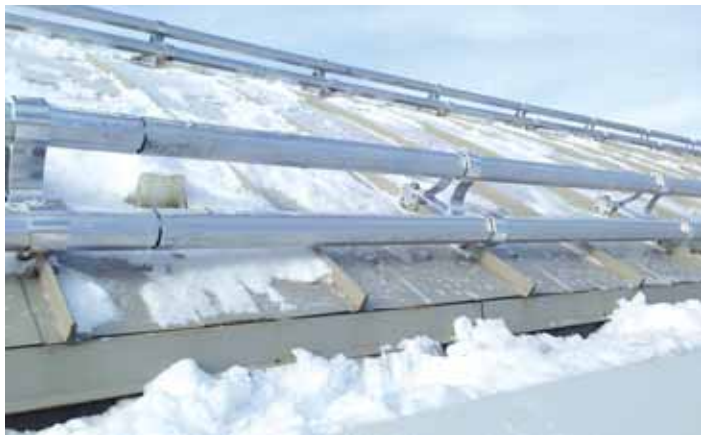
Metal roof snow fence fastens with clamps or brackets. Continuous system attaches near roof eaves.
