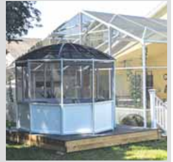
Wood used a 10-ft. dia. satellite dish and 7-ft. poles with vinyl panels to make his gazebo.
