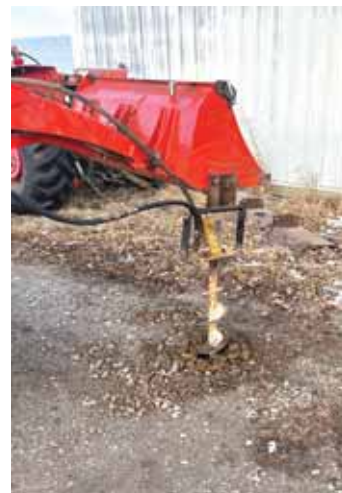
To power the auger, Tschetter disconnected the hydraulic hoses from the tilt cylinder on the loader and connected them to the motor.
