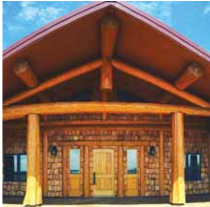
Each house is dry-fitted at the company's work facility before every log is numbered, disassembled, and shipped to the building site.
