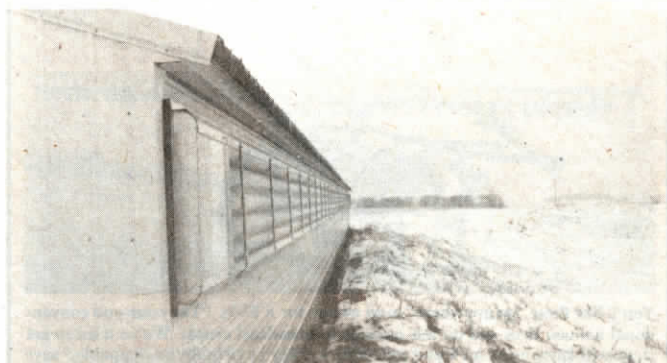
Side ventilation system resembles an air mattress standing on one edge. The air tubes deflate as necessary to let more air into the building.
