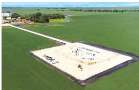
Hiebert's unit is the FP 300 pilot model, which will produce 100 tons of green anhydrous ammonia annually.
