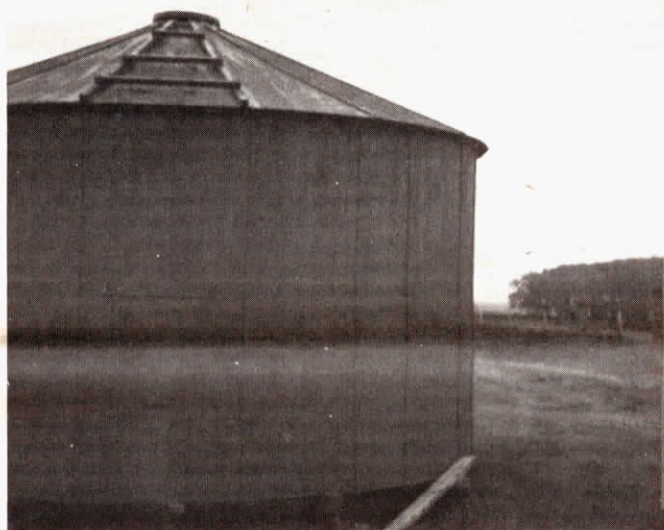
Wood grain bins are built with 3/8-in. plywood. They can be moved easily, if necessary.
