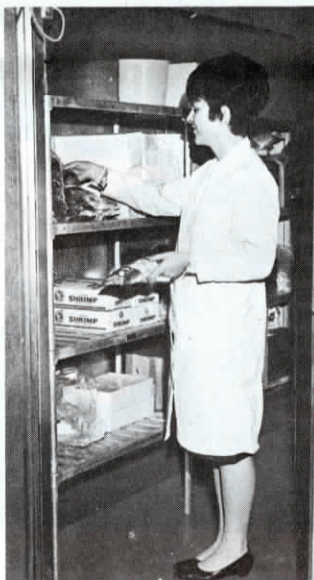
Center aisle is warmed by infra-red heat lamps. Optional shelves for frozen food storage can be installed in place of locker boxes.
