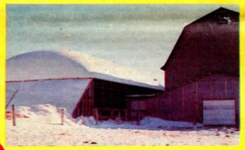
"It's working out great and could well be the silo of the future," says Terrence Weigel, Sr. Giant dome which covers 46 by 65 ft. trench silo cost a lot less to build than a conventional metal or wood roof.
