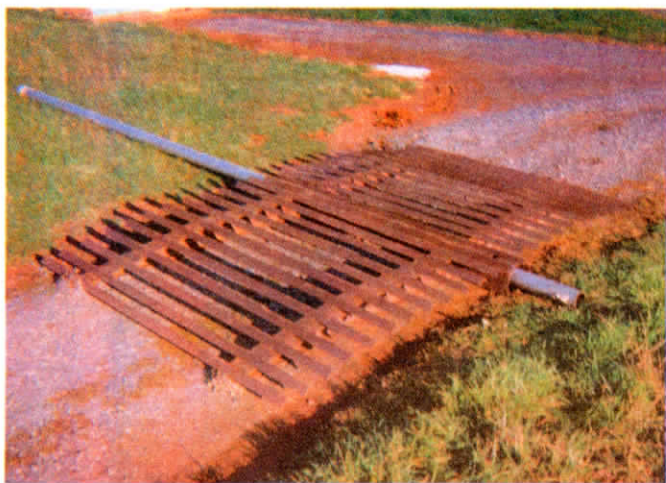
Teates built 6-ft. wide "pipe bridge" from used scrap metal to protect 6-in. dia. pipe that supplies water to his traveling gun irrigation system.
