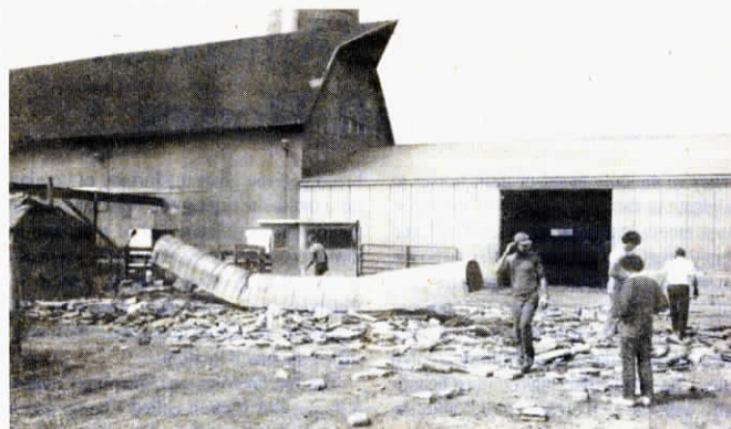
After the silo fell down there was nothing left to salvage - just a big cleanup job.
