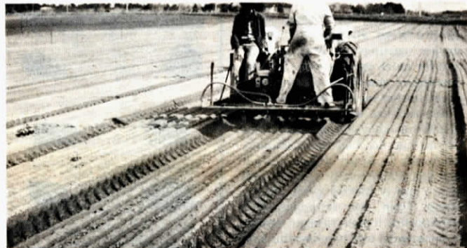
Sprayer applies cement slurry to newly seeded fields.
