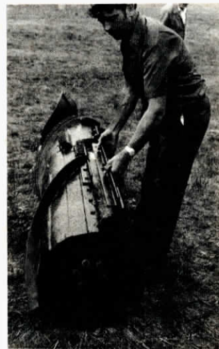
Baxter replaces straight IH threshing bars with curved "helical" bars.
