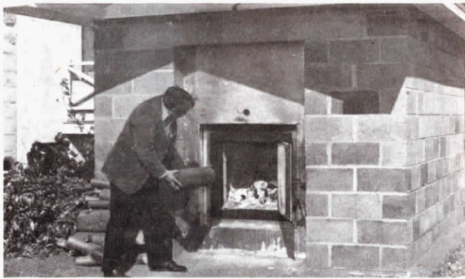
HAHSA is linked to home by underground hot water pipes.
