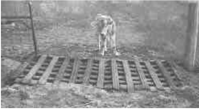
Cattle guard made of 90 20-in. tires costs less to build than conventional.
