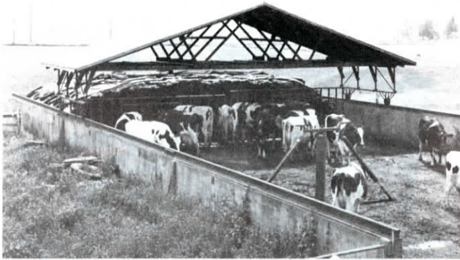
Roof rides on railroad rails mounted on walls of 40-ft. wide bunk silo.
