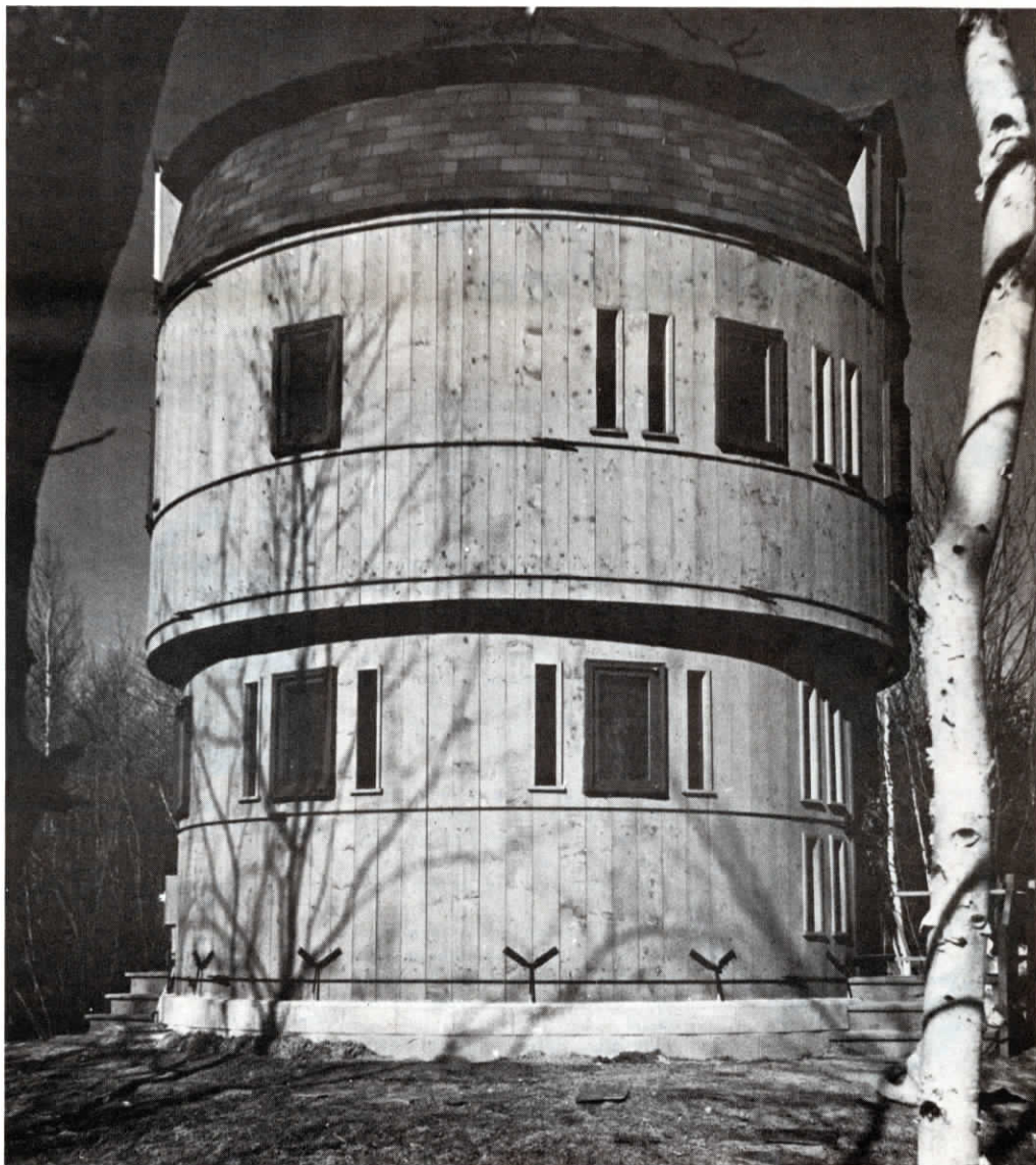
Silo houses are built of 2 in. tongue and grooved wood staves, the same used in building regular silos except that the staves are untreated. Some build two adjacent "silos", with kitchen-dining-living rooms in one, and bedrooms in the other. There is no standard model.
