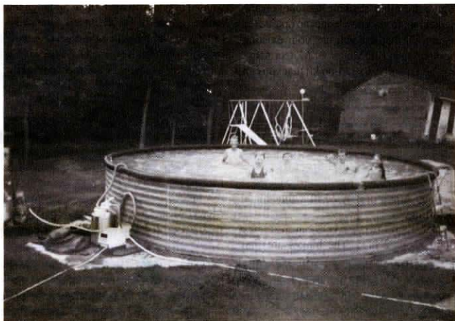
To make the pool, Portner bolted seven bin panels together and sealed them with silicone. He put 3-in. dia. plastic drainage tile, split lengthwise, over the top edge.
