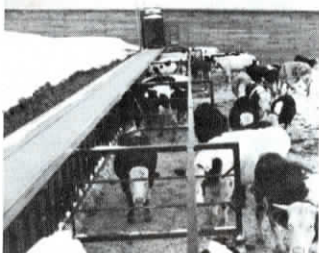
Sides of this bunker silo, equipped with the automatic Bunk Buzzard, are formed by the treated wooden walls of two barns spaced about 100 ft. apart.
