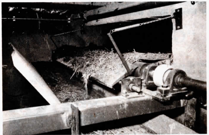
By suspending a net under slats, high value fertilizer solids can be retained while lower value liquids pass through.
