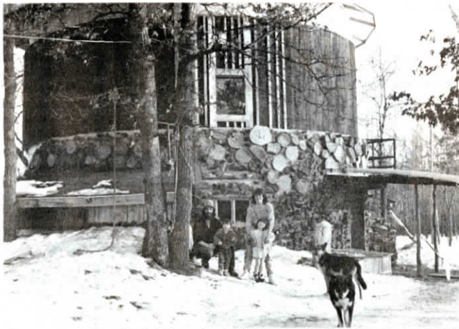
Spear covered the walls of the lower level of the house with 12-in. long cordwood held together with mortar.
