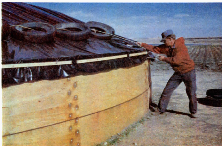
Curtis Hemstad secures 4 by 8 ft. plywood panels with a cable looped around the bin. Plastic top is secured to panelled sides with strips of lath and a ring of tires holds everything in place.
