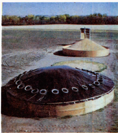
Curtis Hemstad secures 4 by 8 ft. plywood panels with a cable looped around the bin. Plastic top is secured to panelled sides with strips of lath and a ring of tires holds everything in place.
