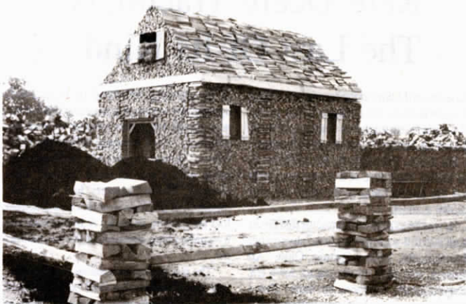
Metker builds a new cabin each year out of 40 to 50 cords of wood.
