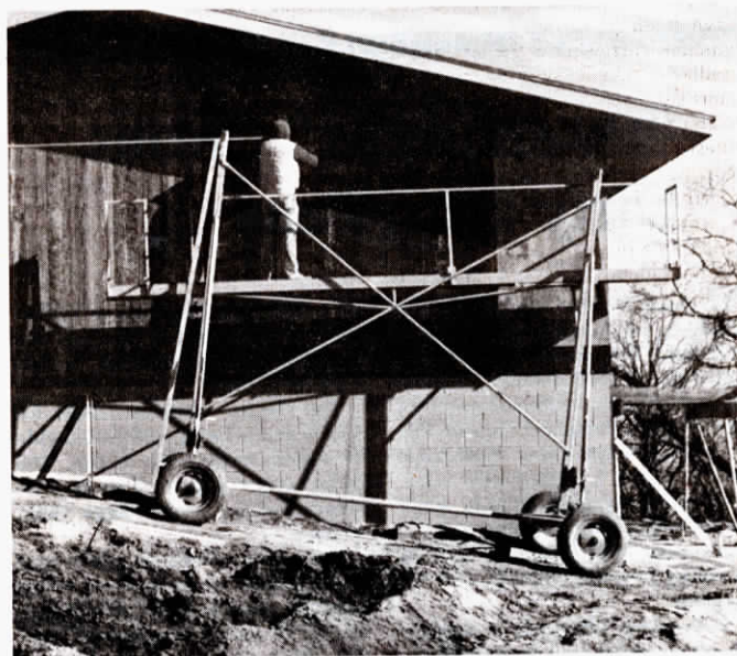
Platform on Rustgo's portable scaffold is leveled at either end with a hand-cranked winch. Folds down for transport in minutes.
