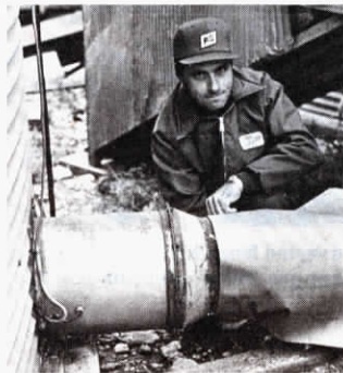
Dave Primus shown at the point where heat is drawn from a cooling bin. He is holding a sheet of paper over the duct to simulate insulation.
