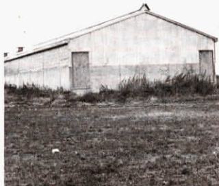
The barn is 36 ft. wide, 90 ft. long and has 27 finishing pens.
