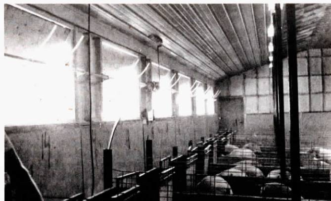
Side doors open, close automatically to let in fresh air as needed.
