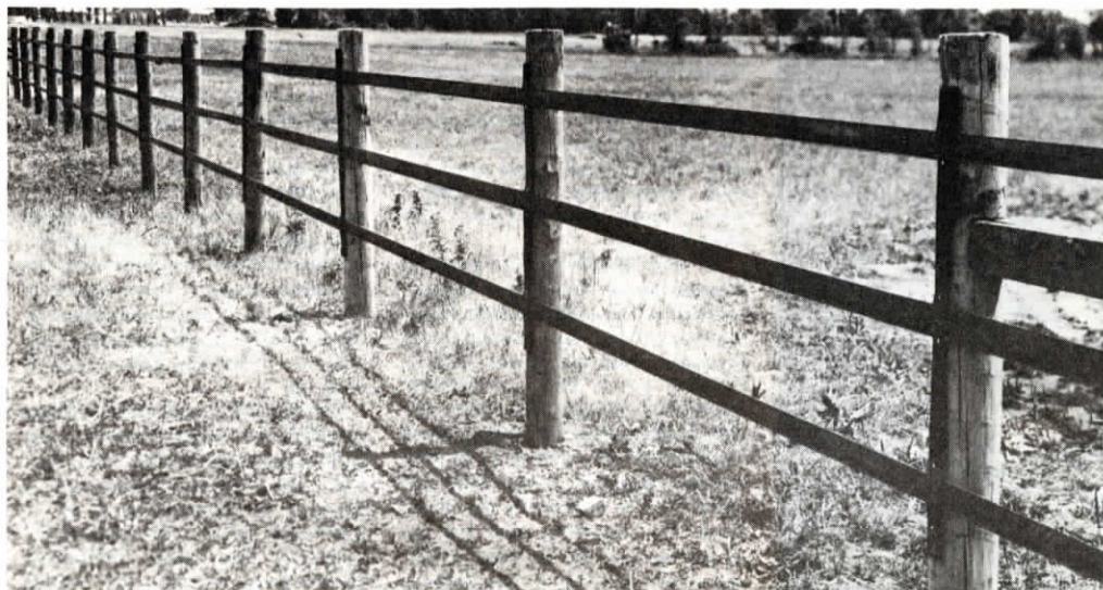
Vertical facing strips used to secure Belt Rail to posts are made from regular belting (4 in. wide) cut in half to make the 2 in. wide strips. Note that nails are above and below the belting at each junction, allowing the horizontal belting freedom to slide back and forth.
