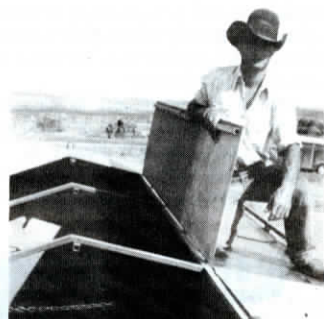
Doors are 2 ft. wide and hinge back, leaving the center open.
