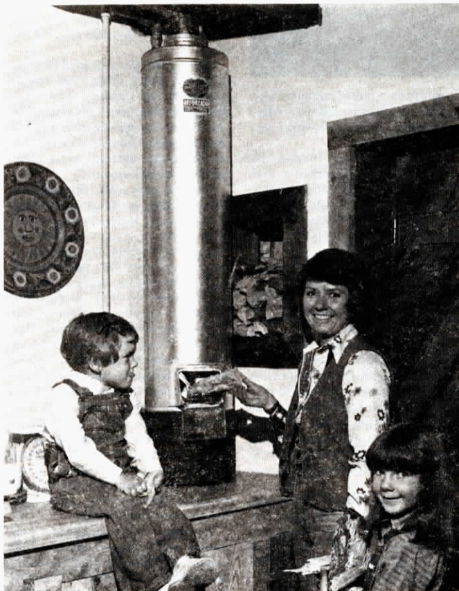
Wood-burning water heater is completely compatible with existing plumbing, according to manufacturer. One model burns used crankcase oil, or kerosene.
