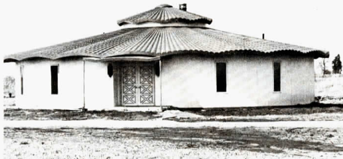
Standard size Concept 21 house is 41 ft. in dia. and provides 1,320 sq. ft. of floor space.
