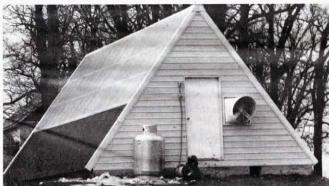
Thompson says the A-frame design wastes less space and is ideal for solar design.
