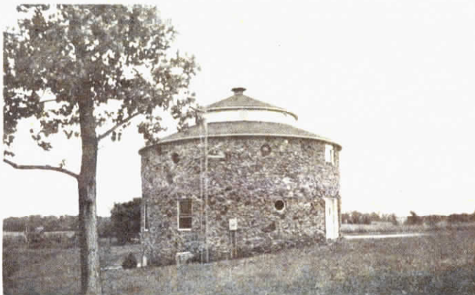
This 4-story, 4-bedroom home was once a 36-ft. dia., 21,000 bu. capacity grain bin.
