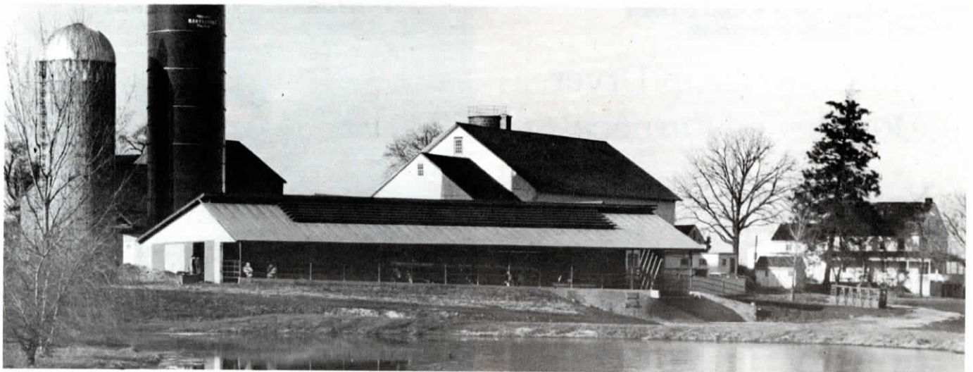
One of some 30 Sol-Air systems which have been installed to date in Pennsylvania and neighboring states.
