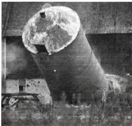
Strategically-placed dynamite charges demolish old silo without damaging barn standing within inches of it!
