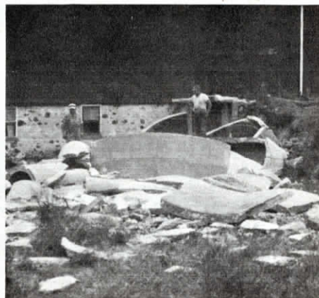
Strategically-placed dynamite charges demolish old silo without damaging barn standing within inches of it!
