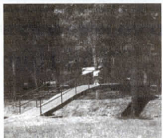
Arched bridge across creek is 53-ft. long.
