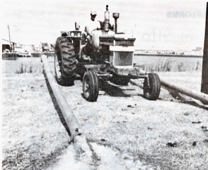
Home-made rig, which cost $300 to build, can pump up to 5,000 gal./min.
