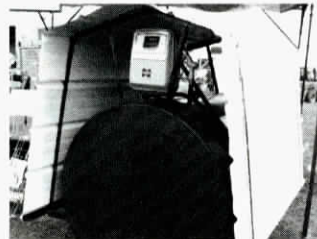
White corrugated metal sheets are pre-formed to create shelter's barn-roof shape.
