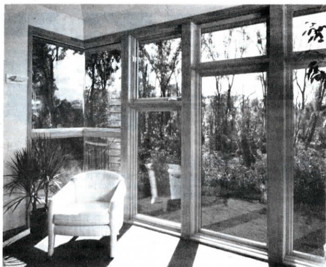
Window makes the turn around corners with no structural member to block view.
