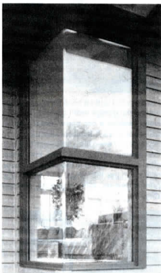
The two panes of glass make a 90° turn without any seam at the corner joint.
