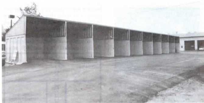
Compartmentalized "commodity sheds" form bins 8 1/2 ft. high, 12 to 14 ft. wide.
